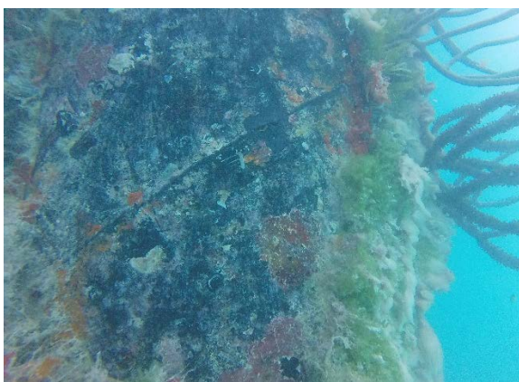
Fig. 2c 2 nd Level 2 inspection, Pile 165
