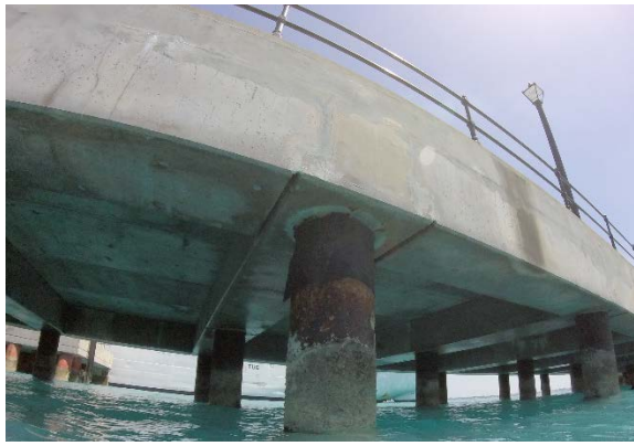
Fig. 2e – General view of Gangway splash zone
