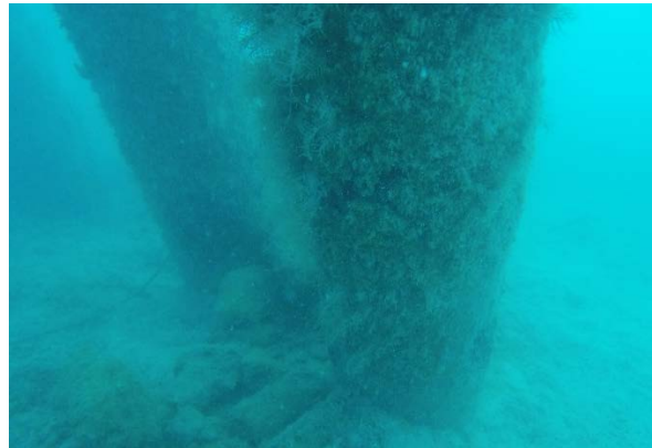
Fig. 3n Piles driven into sandy bottom, H-MD3
