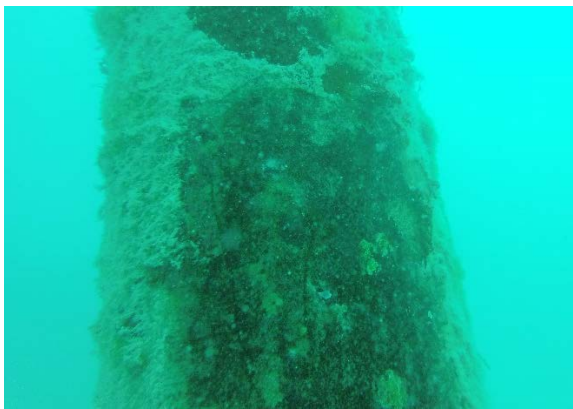
Fig. 3q - 1 st Level 2 inspection, walkway dolphin
