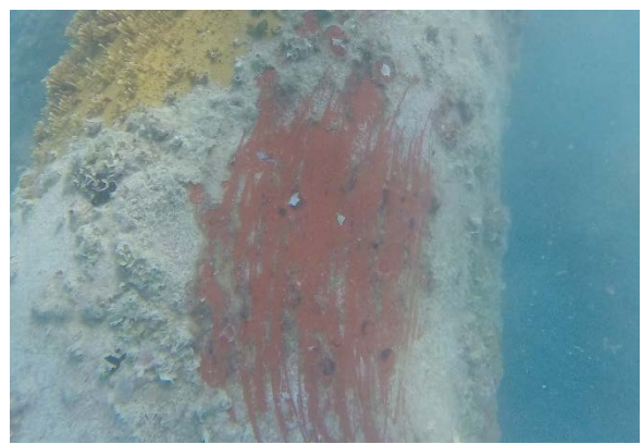
Fig. 3f - 2 nd Level 2 inspection, HMD6
