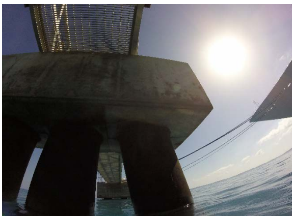
Fig. 3o General view of walkway dolphin
