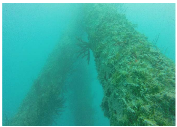
Fig. 3p General underwater view of original walkway dolphin piles
