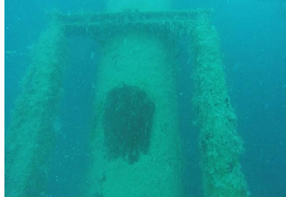
Fig. 3t – Anode and Level 2 inspection on H-BD3
