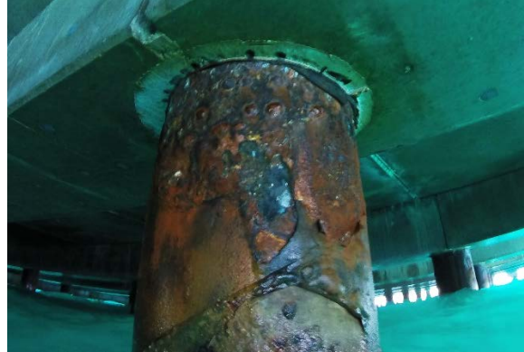
Fig. 1q Top of pile of Cluster 2
