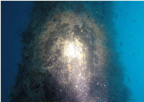
Fig. 1l 1 st Level 2 inspection, Pile 45, protective coating intact
