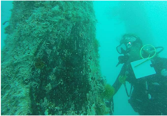
Fig. 3y - Level 2 inspection at middle of pile, H-MD2, protective coating intact
