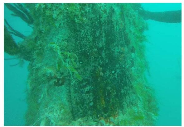
Fig. 3r - 2 nd Level 2 inspection, walkway dolphin
