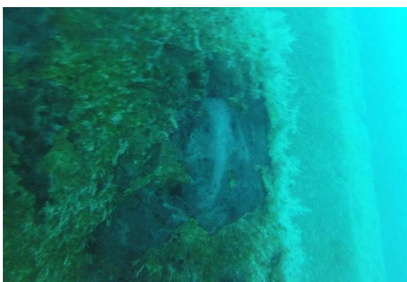
Fig. 2i - Level 2 inspection on sheet pile to probe ALWC depth
