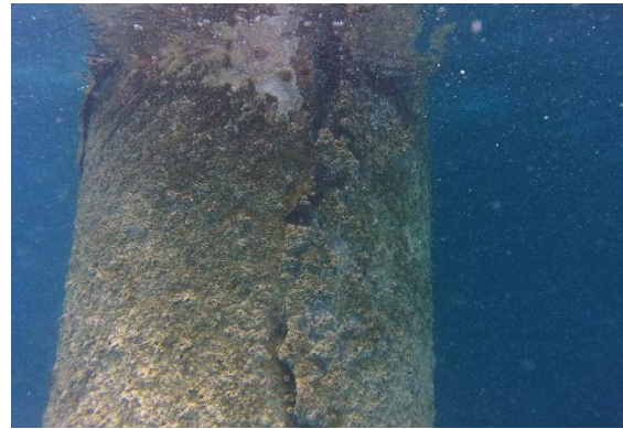
Fig. 1w – Just below surface, Pile 66
