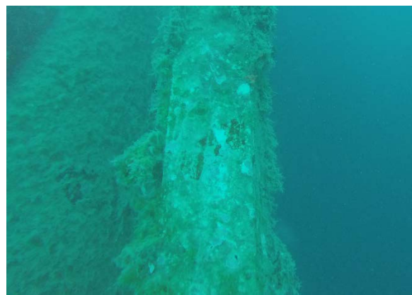
Fig. 3v - Level 2 inspection on anode, H-BD3
