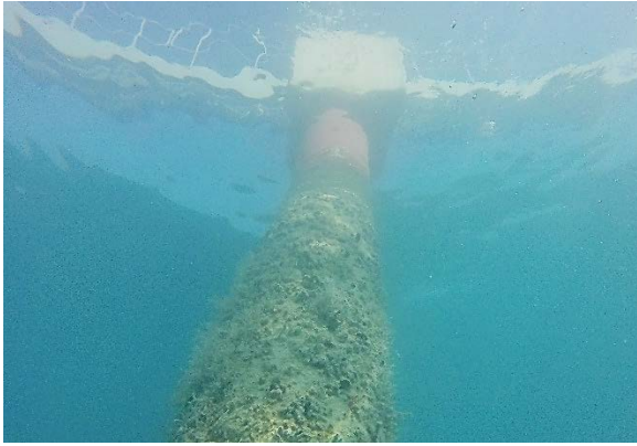
Fig. 3g - One of the three piles on walkway dolphin
