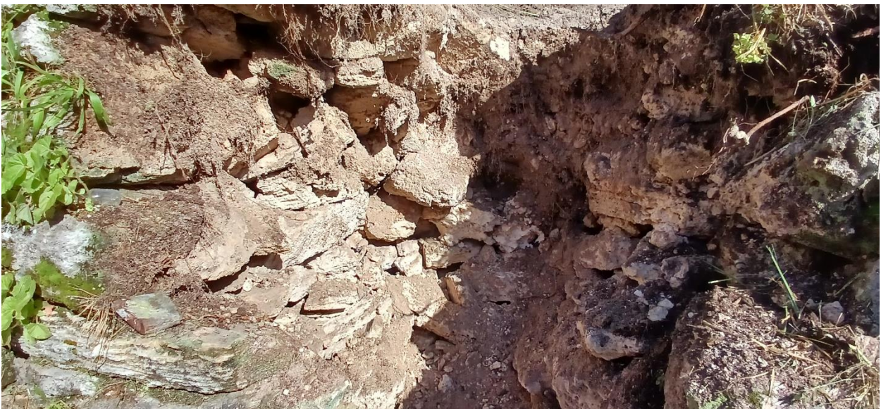
Figure 3 - Close up view of investigation. Only fill material found.
