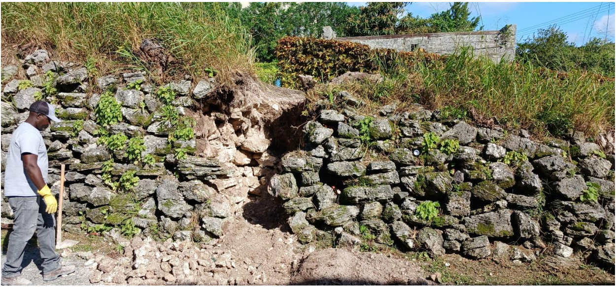
Figure 1 - Intrusive investigation into dry-stone wall
