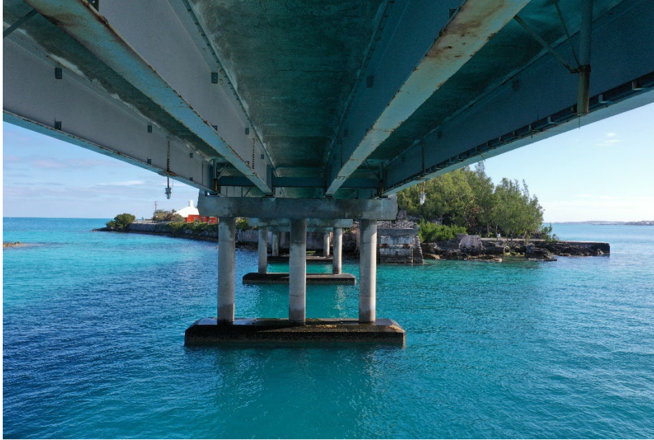
Photograph 13 – Span 4 Main Girders.
