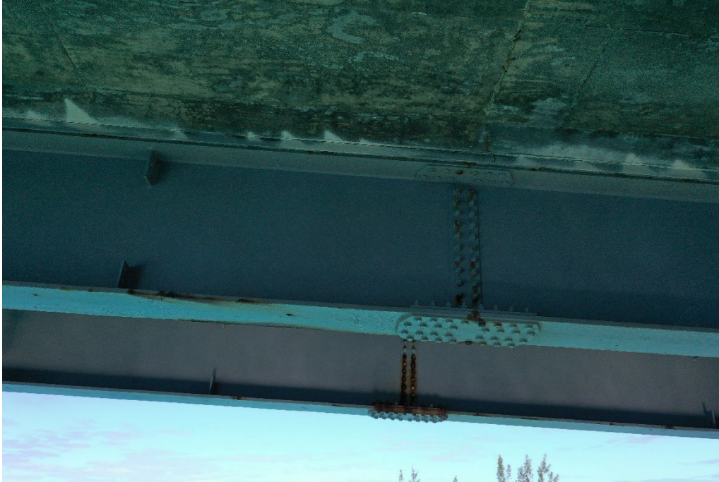
Photograph 17 – Span 7 Main girders and splice connections.
