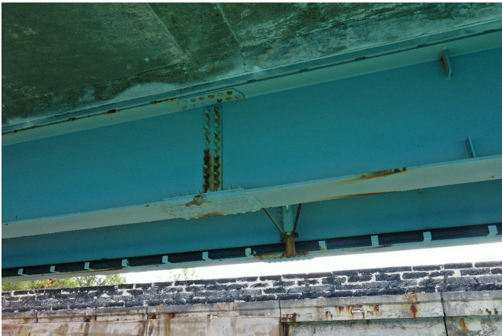
Photograph 18 – Span 7 Main girders and splice connections(1).
