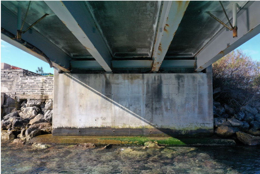
Photograph 1 – Abutment A1 – Elevation.
