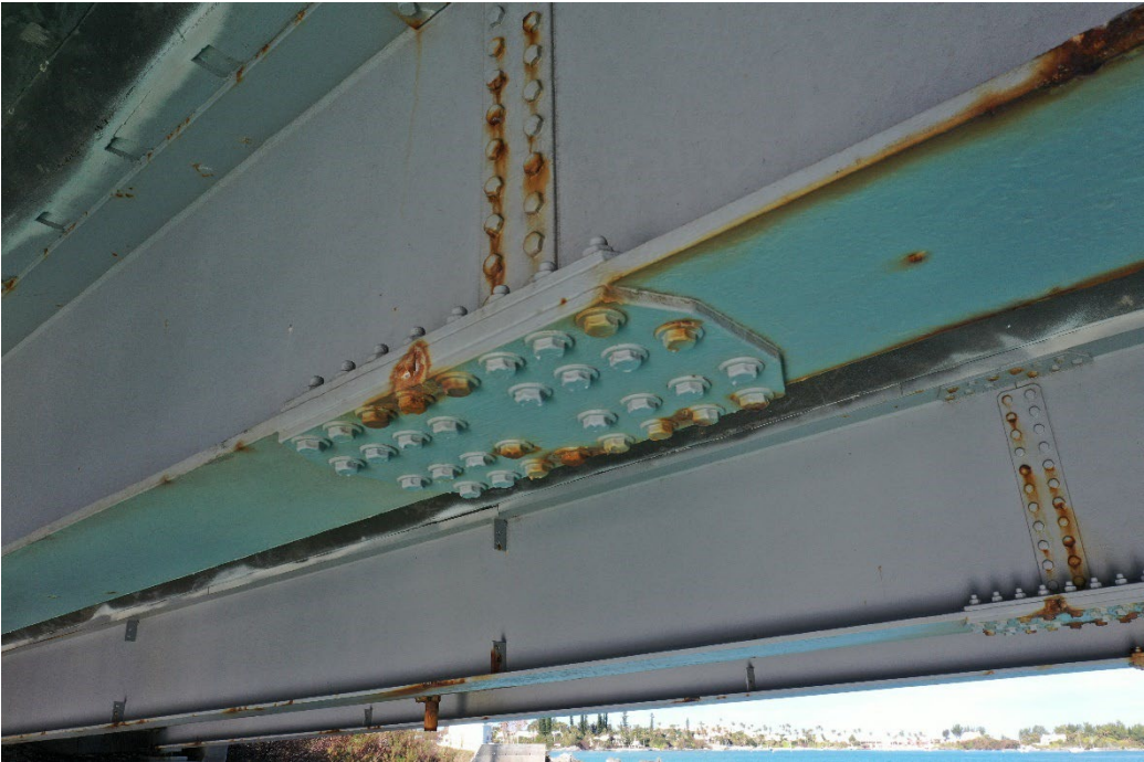
Photograph 3 – Span 1 Plate girder splice connection.
