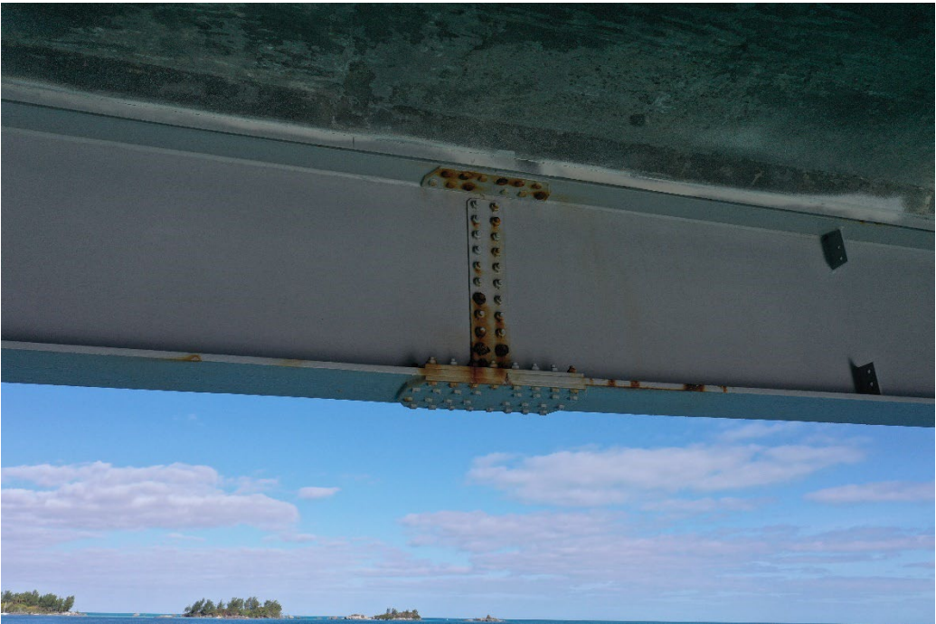
Photograph 4 – Span 1 Plate girder splice connection (1).
