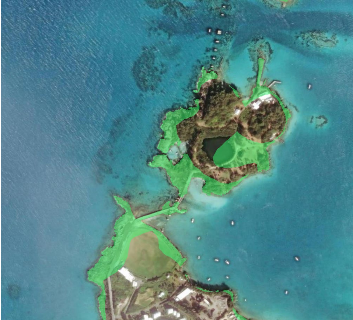
Figure 9.21 Coney Island Bridge affected by saltwater inundation during the SSP5-8.5 100yr scenario (Note: data is not shown for suspended bridge deck sections).
