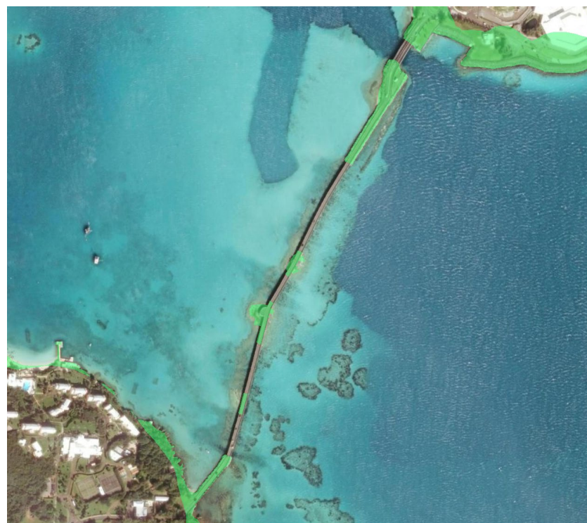
Figure 9.12 Causeway/Longbird Bridge affected by saltwater inundation during the SSP5-8.5 100yr scenario (Note: data is not shown for suspended bridge deck sections)
