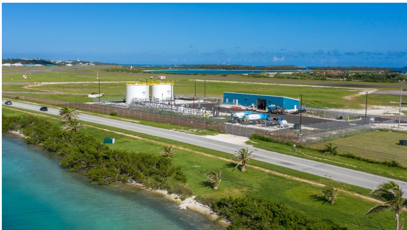
Figure 9.7 Sol Fuel Storage and Supply Facility (OBMI, 2024)
