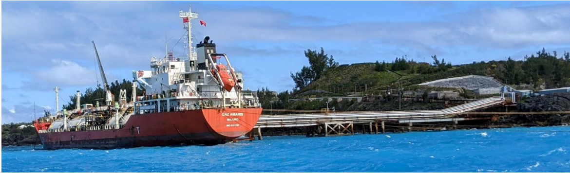
Figure 9.32 Oil Docks Pier
