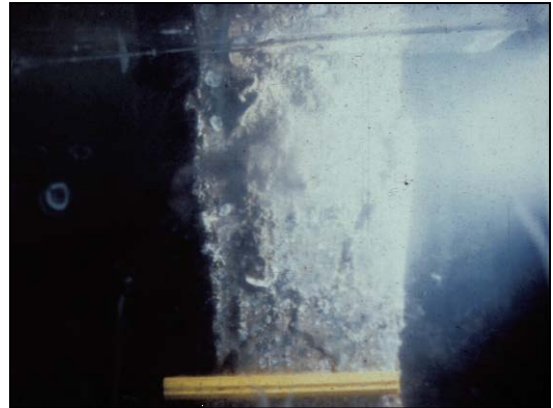
Figure 3-21 Cracked Concrete Pile
