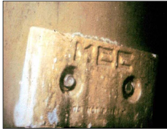
Figure 3-33 Sacrificial Anode on Steel Pipe Pile
