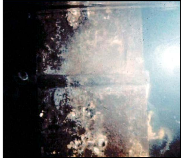
Figure 3-31 Welded Splice of H-Pile
