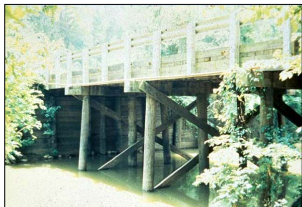
Figure 3-3 Timber Pile Bents and Timber Pile Abutment
