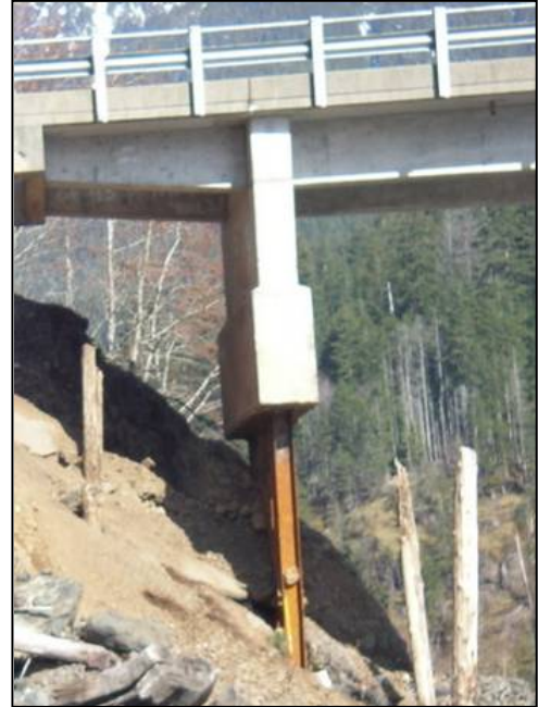
Figure 3-6 Concrete Pier Supported by Steel H-Piles
