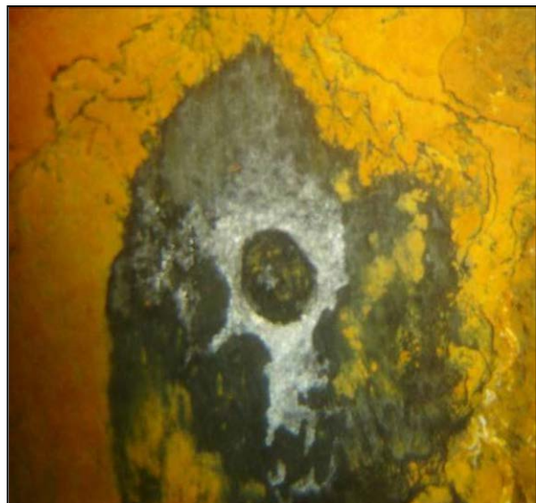
Figure 3-29 Steel Sheet Pile with MIC
