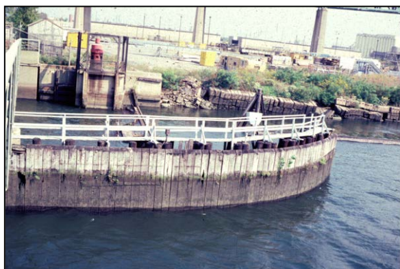
Figure 3-19 Timber Shear Fence
