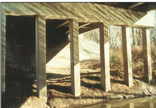
Figure 3-2 Concrete Pile Bent at Low Water
