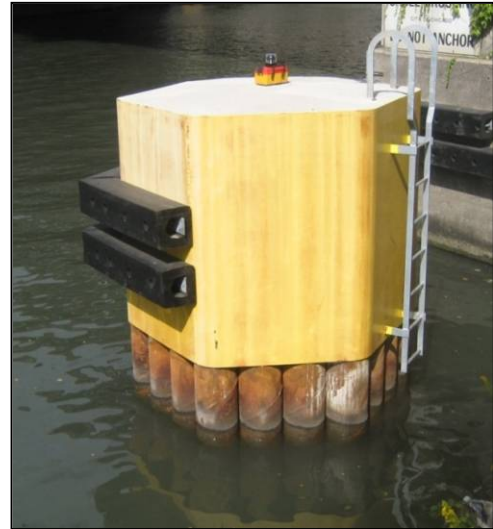
Figure 3-16 Steel Pipe Pile Dolphin with Concrete Cap
