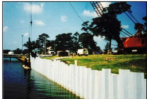
Figure 3-9 Composite Sheet Piling
