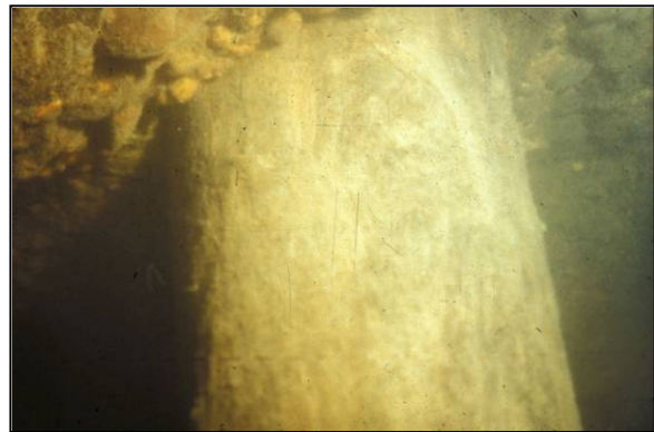
Figure 3-5 Timber Pile at Underside of Concrete Pier
