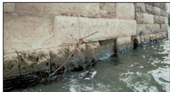
Figure 3-34 Masonry Bridge Pier of Two Types of Stone
