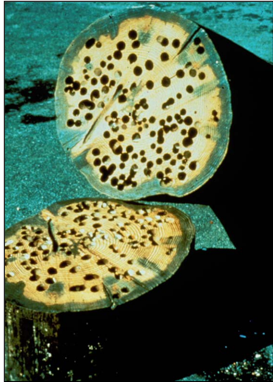
Figure 3-36 Timber Pile with Teredo Damage
