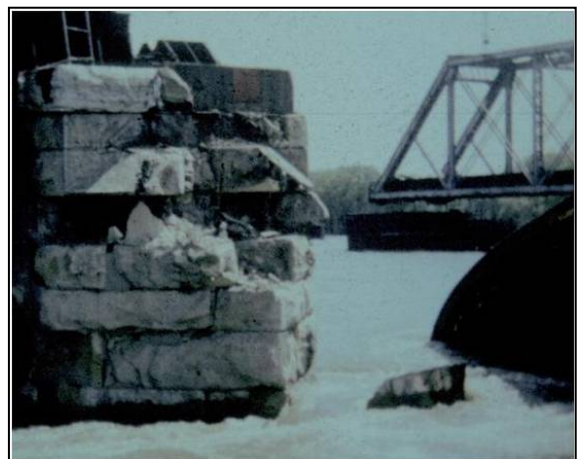
Figure 3-41 Vessel Damage
