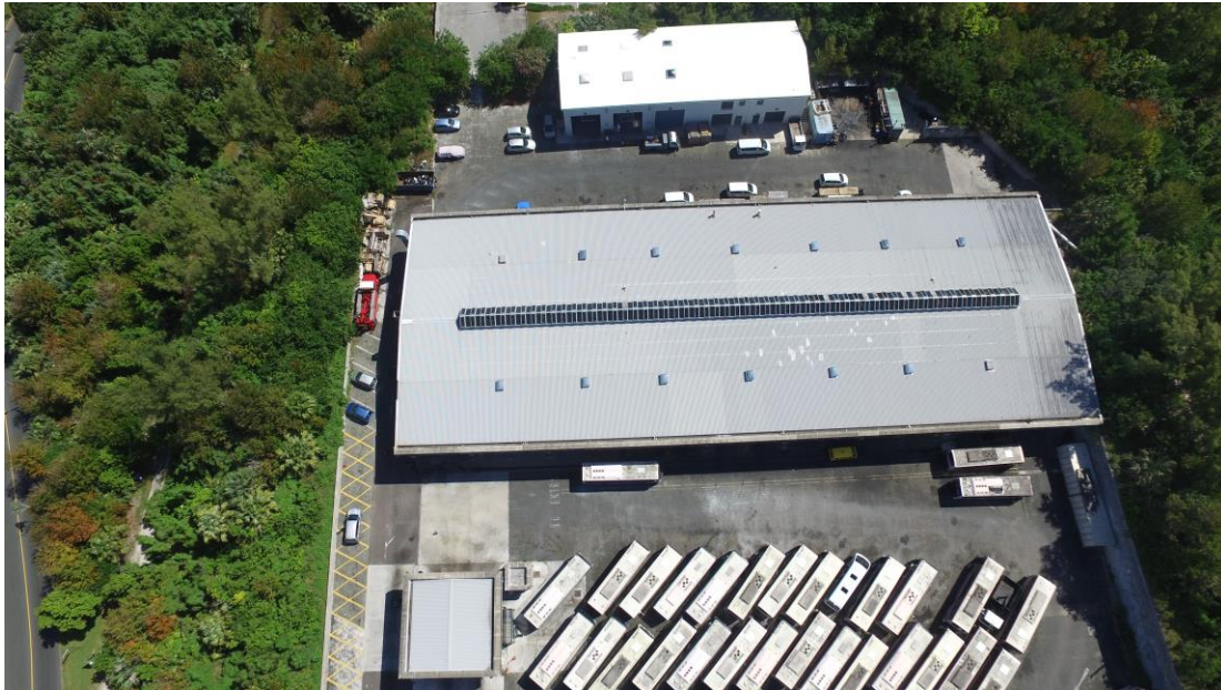
Public Transport Board Garage Roof
