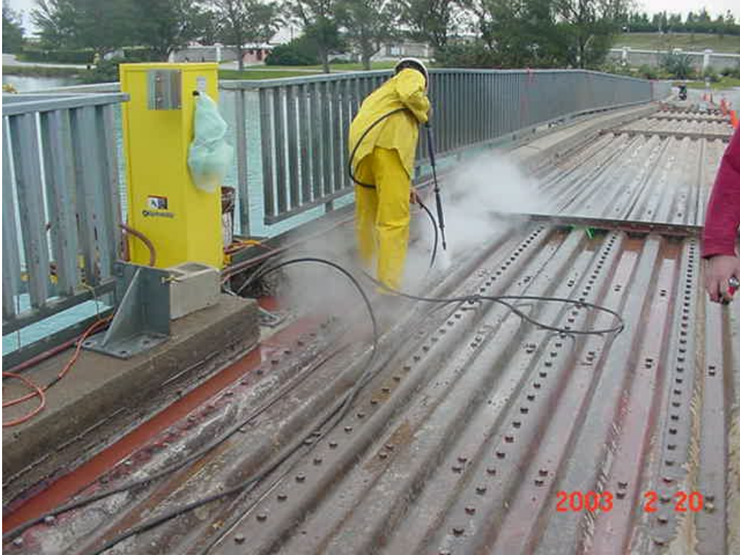
Photograph 5 – Deck cleaning
