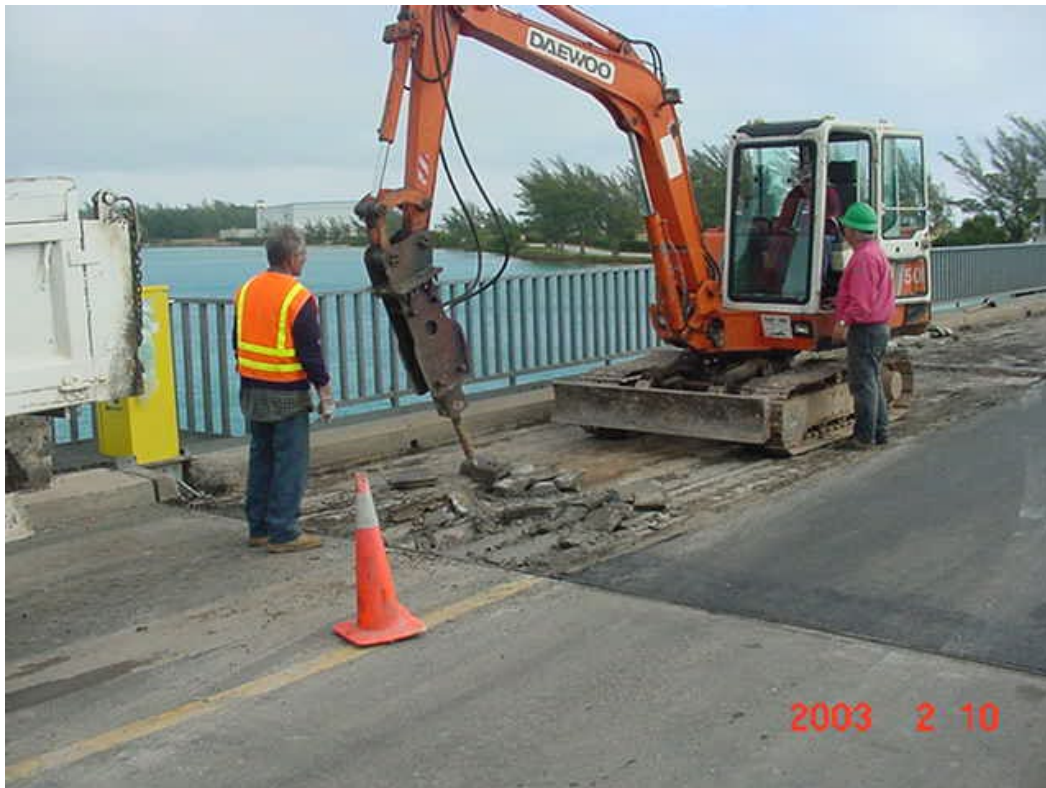
Photograph 2 – Excavator removing concrete from troughs
