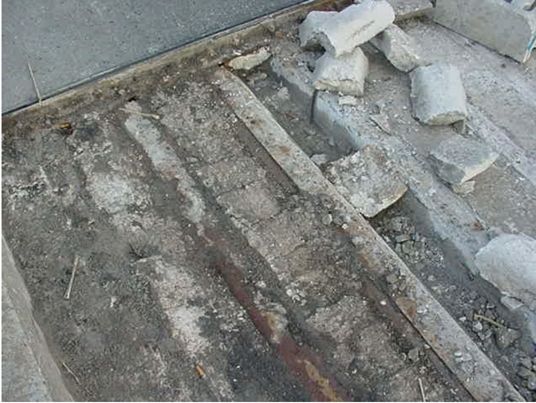
Photograph 3 – Chunks of concrete during removal, approx. 8" long
