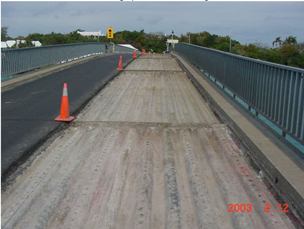
Photograph 6 – Bare troughing
