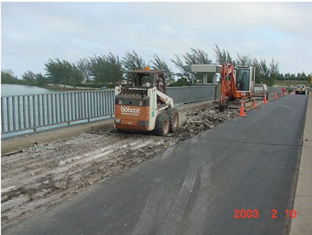
Photograph 4 – Concrete removal
