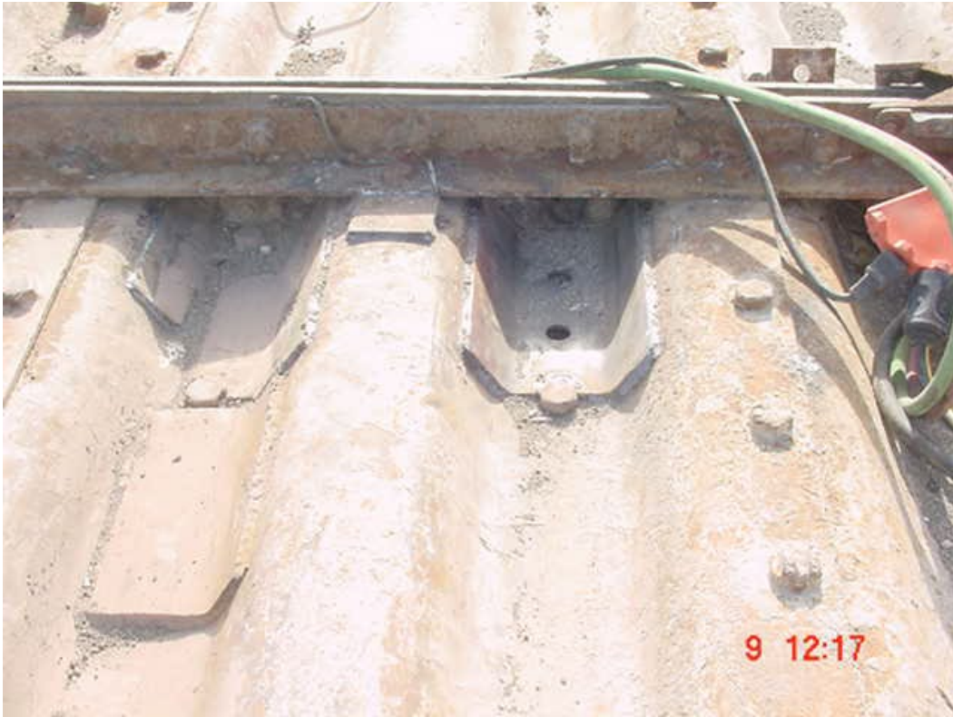
Photograph 7 – Span end plates
