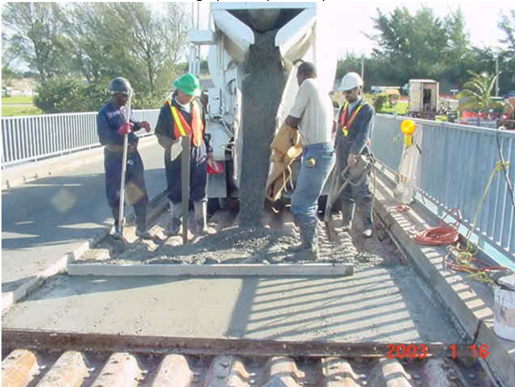
Photograph 8 – Concrete reinstatement
