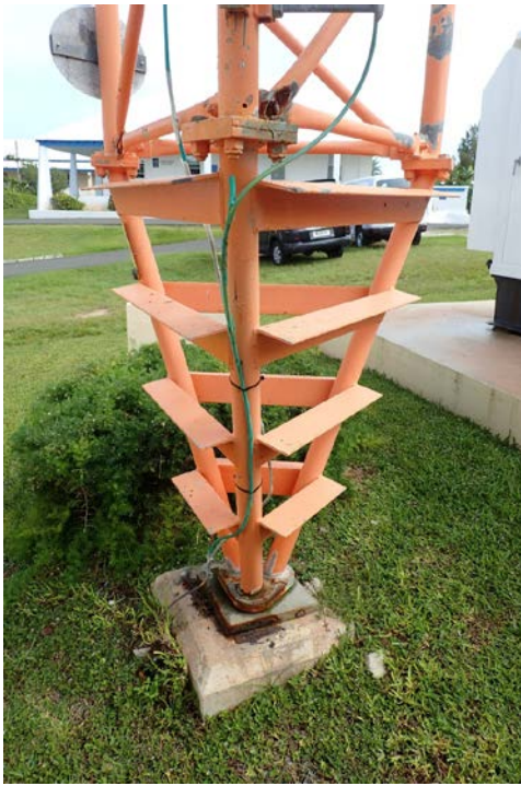
Base of tower File 009
