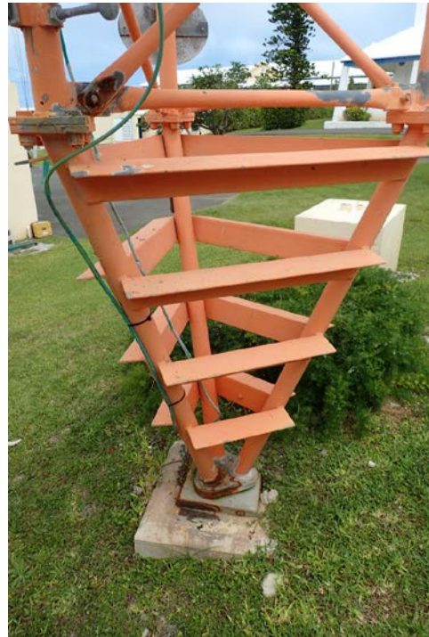
Base of tower File 040
