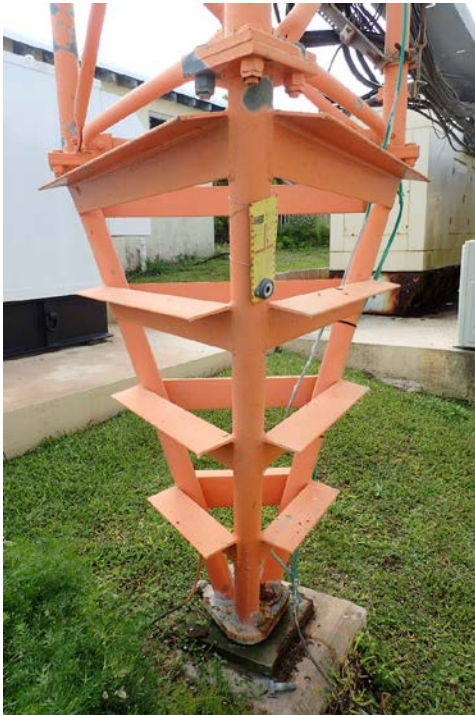
Base of tower File 003
