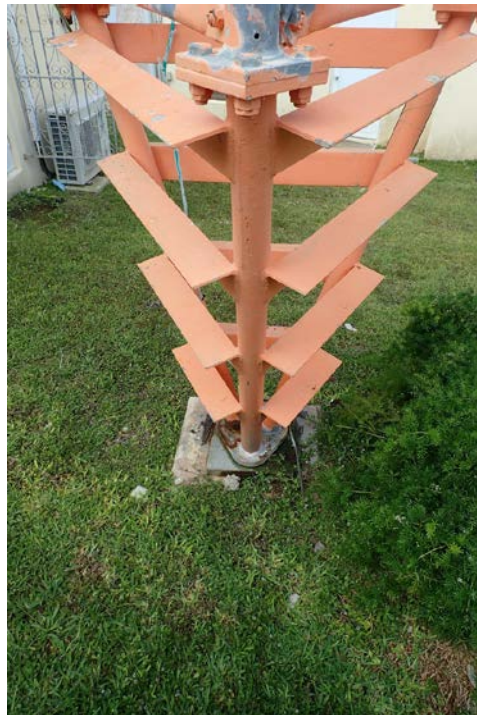
Base of tower File 006
