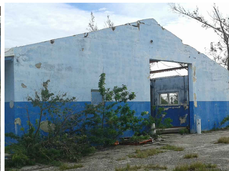
SIDE VIEW OF ATTACHED BUILDING
