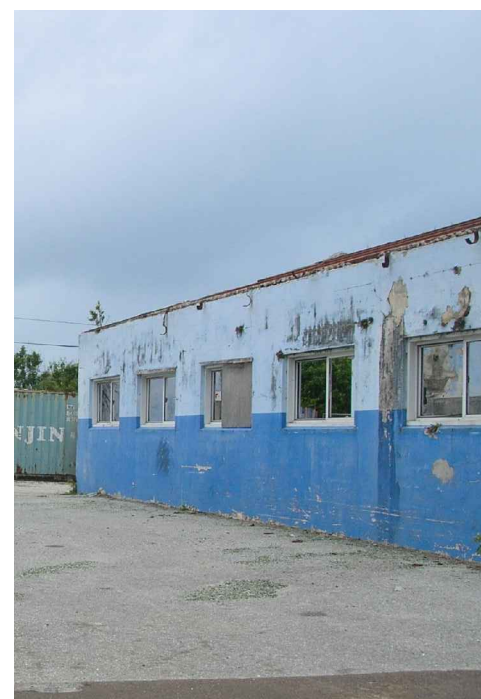
REAR VIEW ATTACHED BUILDING
