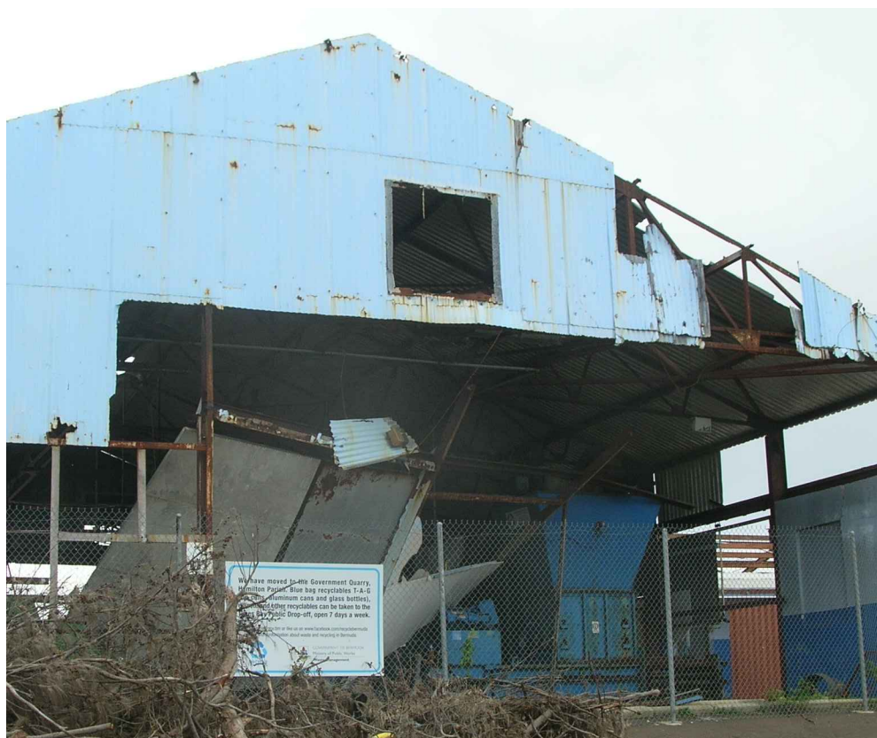
FRONT VIEW OLD RECYCLING PLANT
