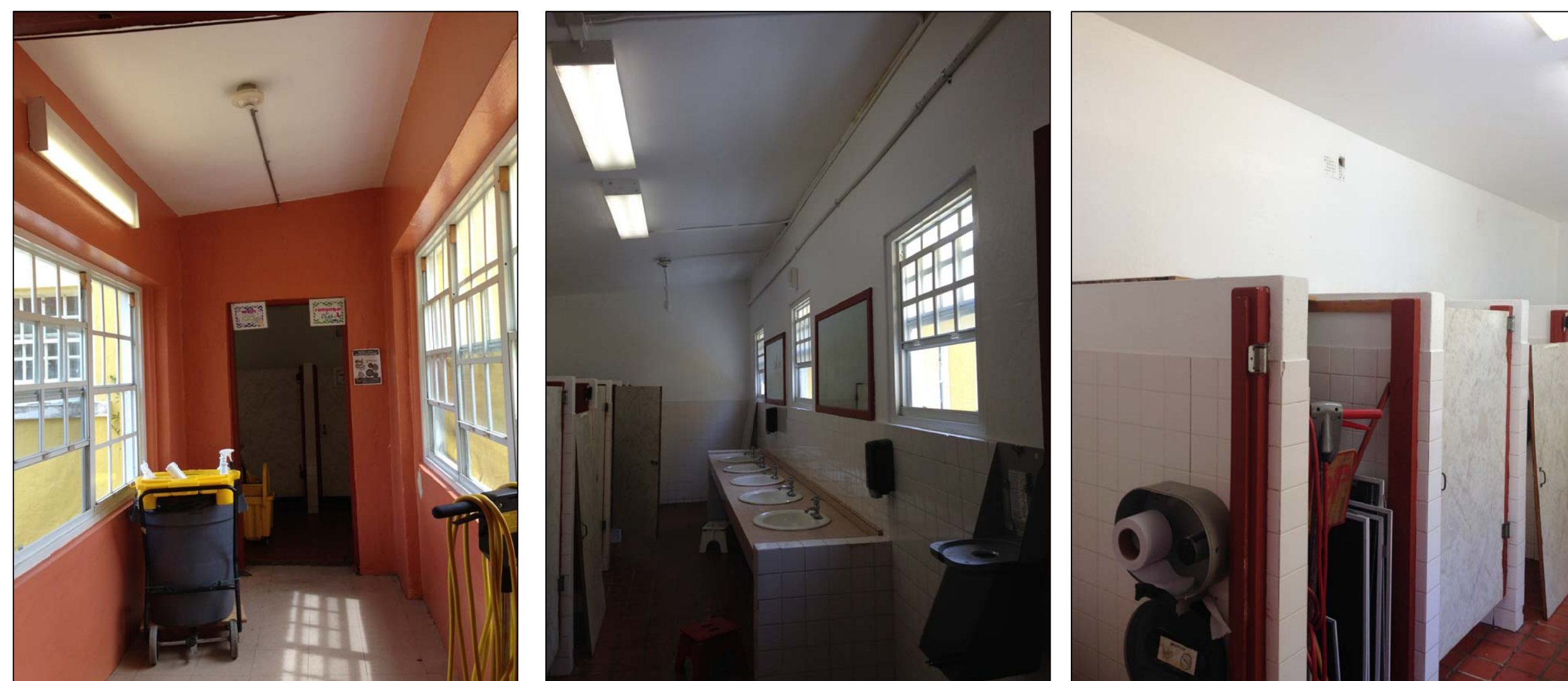
2 Existing Photos of Girls' Bathroom NTS
